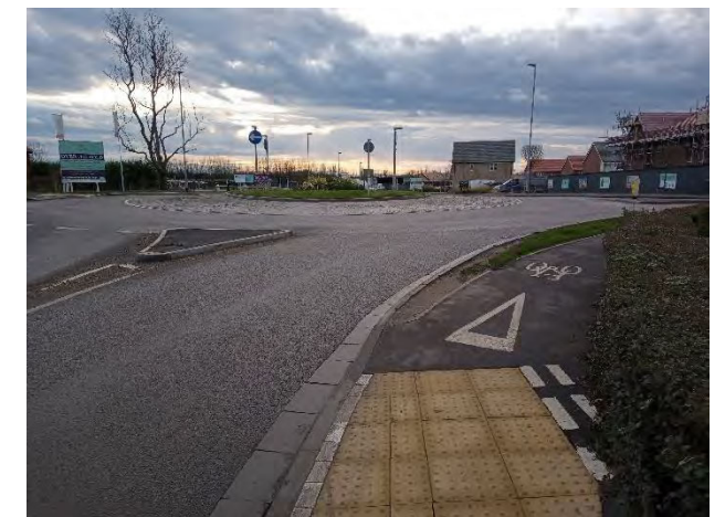
The preferred alignment would enter/ exit Fordham via the new development at Rayner's Green. Unfortunately the new infrastructure is not LTN1/20 compliant and will need changing to bring it up to standard. (The shared use path above is an example)
